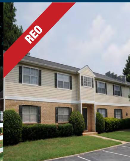
Oaks at Stonecrest, Lithonia, GA 280 Units, built in 1971 $5,400,000 $19,286 per unit
